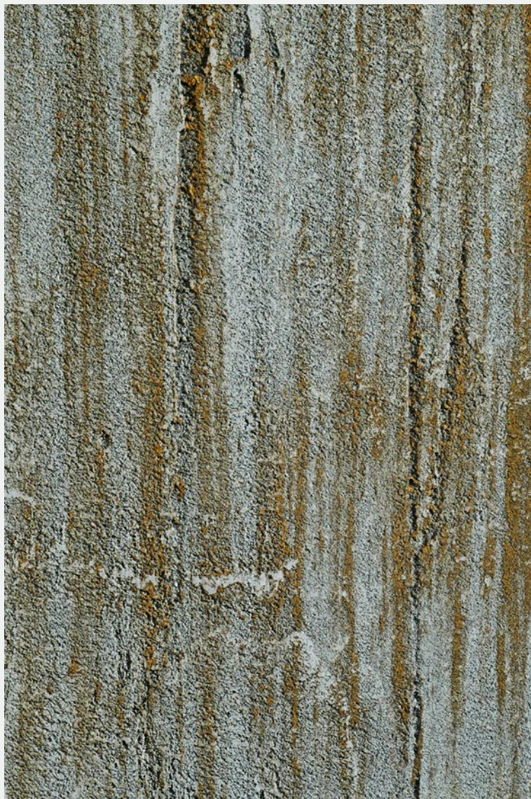
CONCRETE BY NOVACOLOR 17008 & IRONIC & FASE SILOSSANICA 6101
